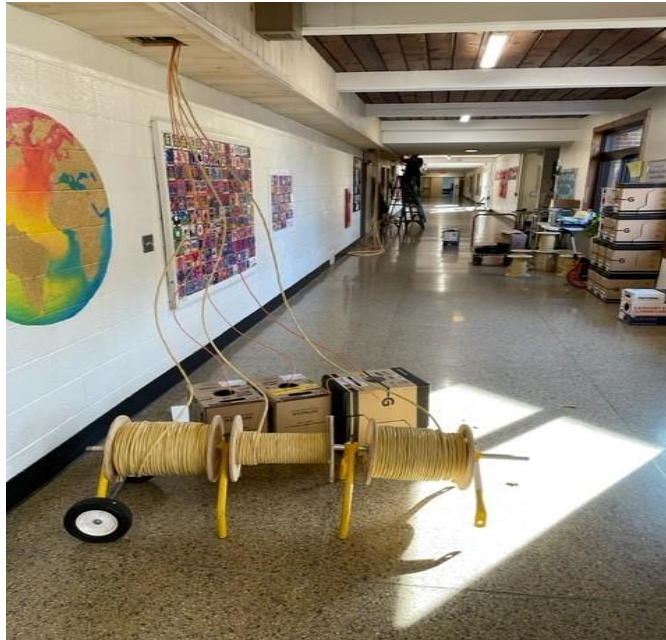
Smithtown Districtwide New Door Installation and Gateway installation to activate doors
