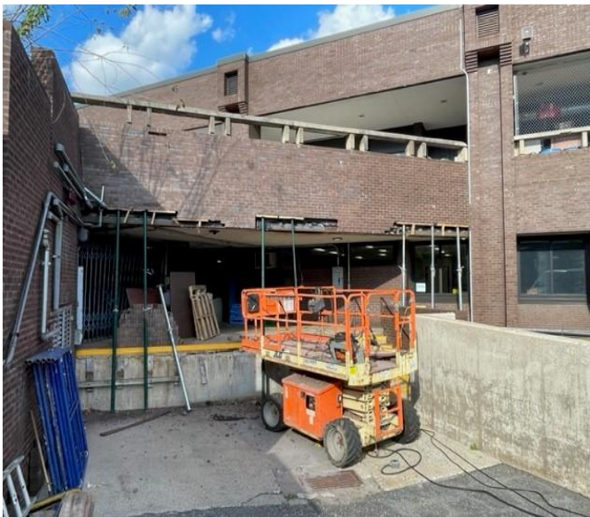
New FRP Doors at HSW in progress , new blind installation at St James Elementary School and new lintel installation in progress at loading dock at HSW
