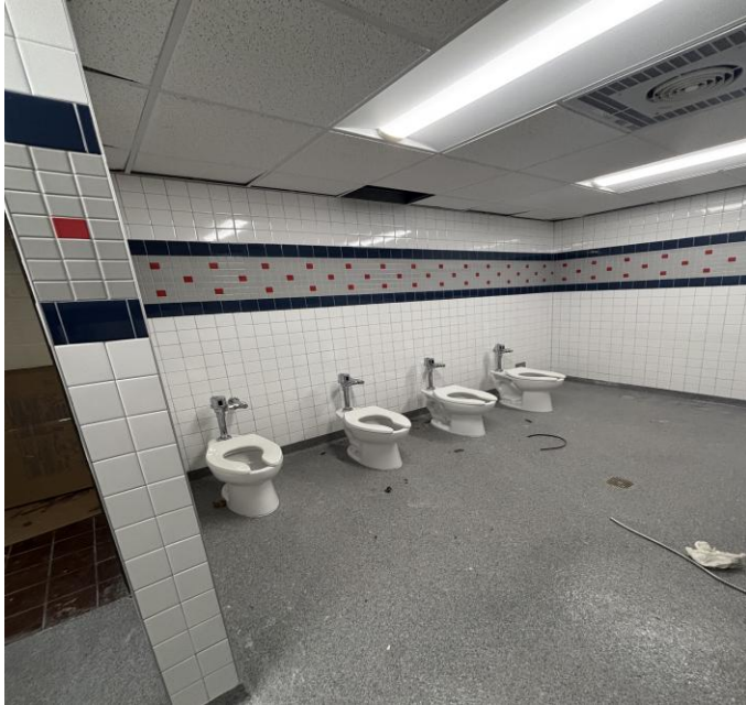
Plumbing fixtures and toilet accessories installed at toilet rooms.
