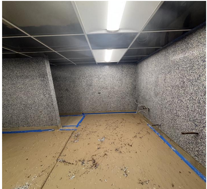
Epoxy wall finish applied to walls at Mt Pleasant ES toilet rooms.
