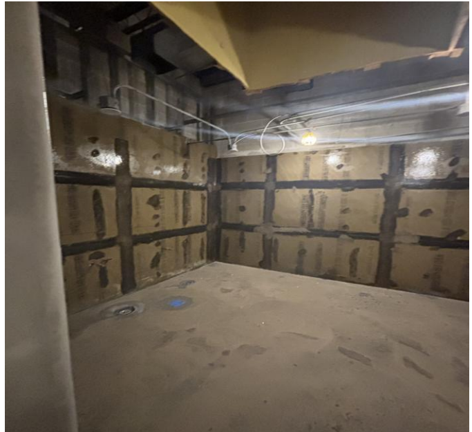
Application of epoxy wall primer completed at Mt Pleasant ES toilet rooms.
