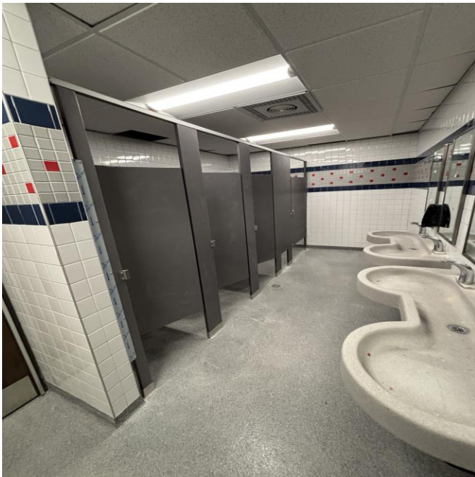
Toilet partitions installed at toilet rooms.
