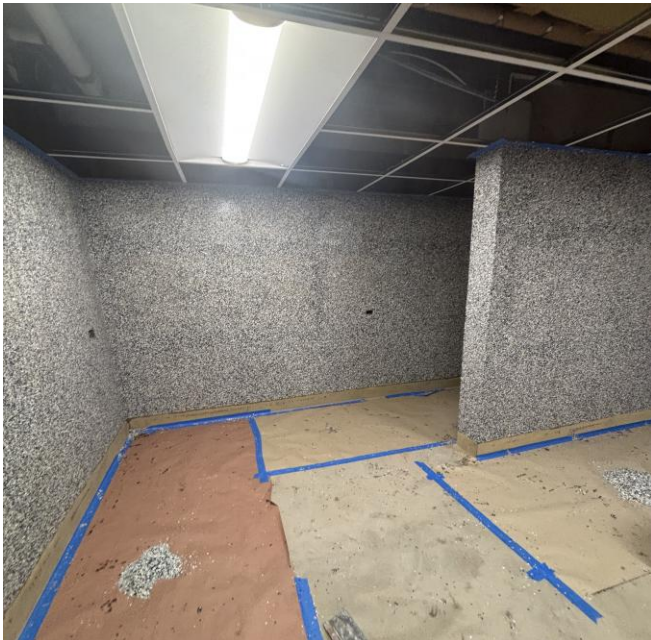
Epoxy wall finish applied to walls at Mt Pleasant ES toilet rooms.
