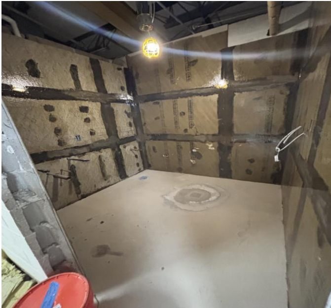
Application of epoxy wall primer completed at Mt Pleasant ES toilet rooms.
