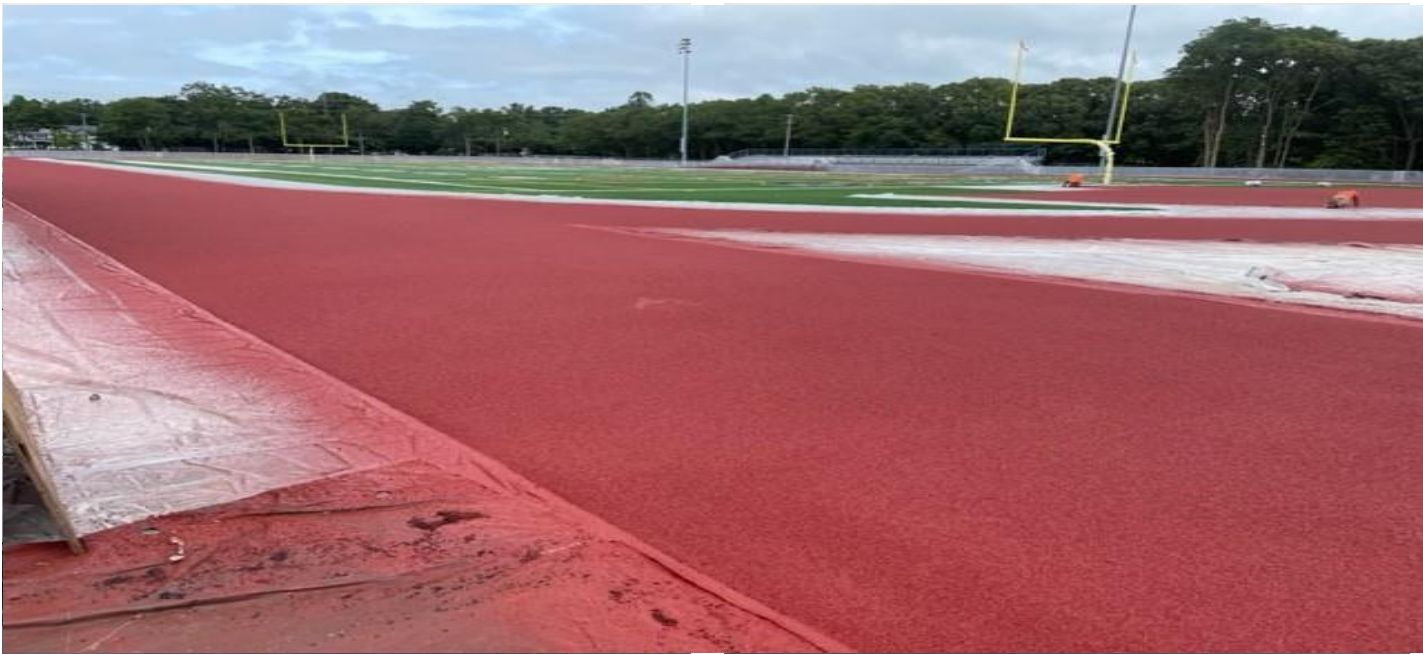
New track installation at Smithtown High School West
