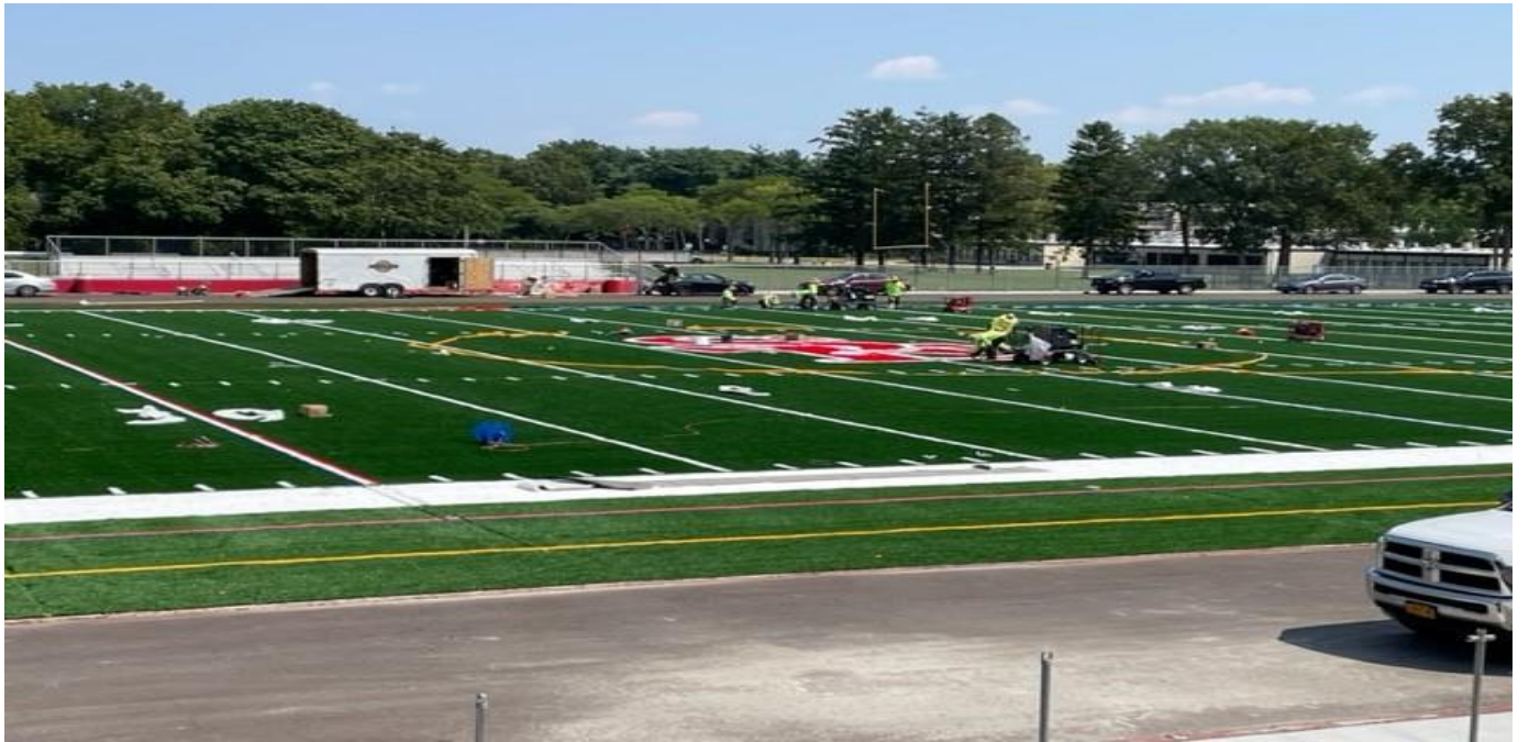
New field turf at Smithtown High School East football field
