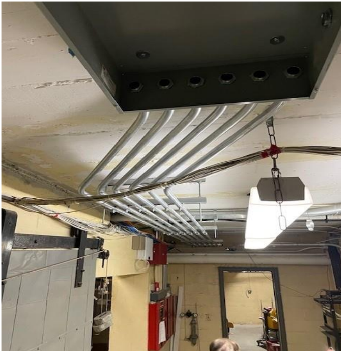
St James Elementary School Unit Ventilation project rough progress - re-routed ductwork and new electrical feed installation
