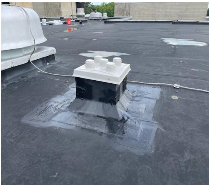
High School East Conduit installation for new Unit Ventilation project, Copper installation in FACS area, and Roof curbs on upper roofs installed
