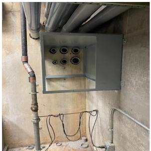
High School East Conduit installation for new Unit Ventilation project conduits and pull box installations
