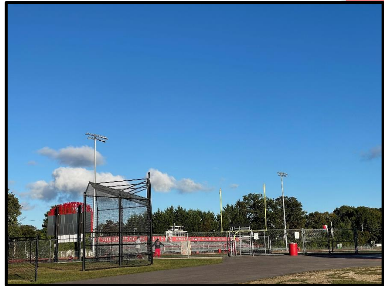
New Stadium Field Lights
