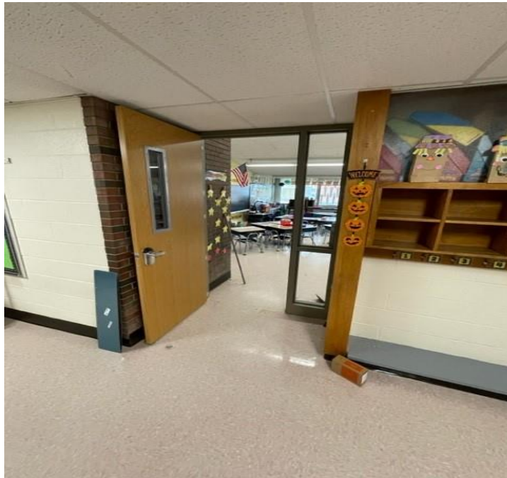
Smithtown Districtwide New Door Installation continues- above are pictures from Mills Pond Elementary School installation
