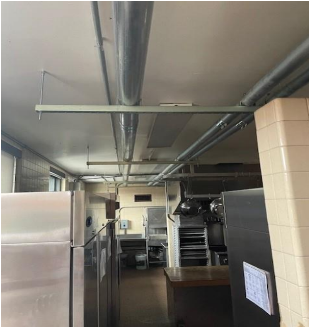
Smithtown Elementary School new conduit installation in progress for the Unit Ventilator project
