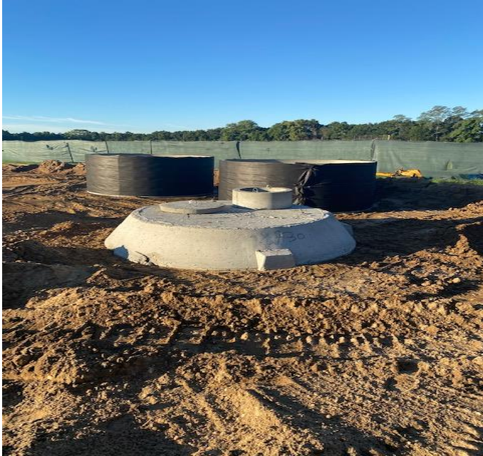
Storm drywell systems installed in foul territory outside field of play to collect storm water at softball field and baseball fields.
