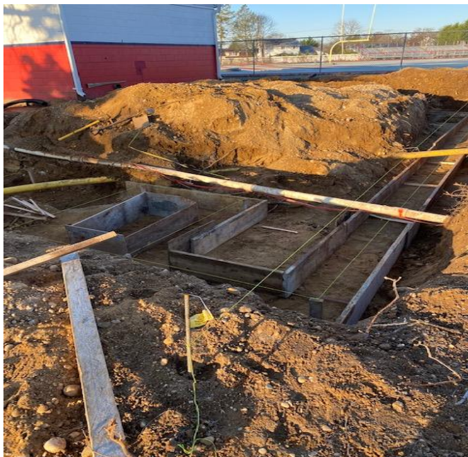
Excavation for the Fieldhouse addition commenced at High School East. Footings are formed and awaiting concrete pour.
