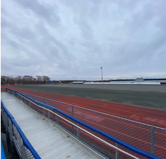
Removal of existing synthetic turf completed at stadium field. Additional gravel fines installed as required.
