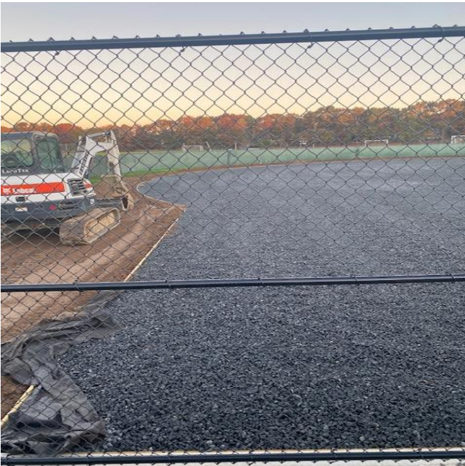
Upon establishing subgrade, gravel fines installed over flat pipe drainage system. Awaiting synthetic turf install.
