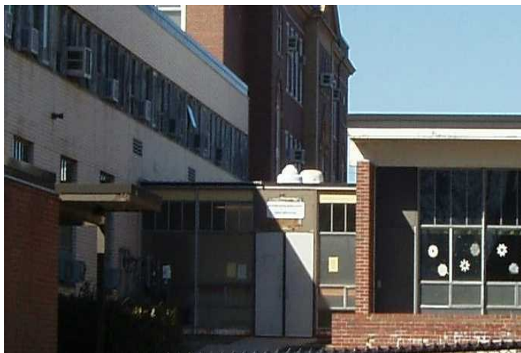
New York Avenue Annex, Joseph M. Barton District Building
