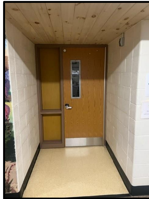
Smithtown Elementary Door Replacement
