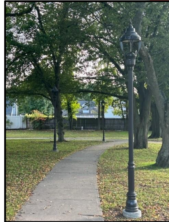
Smithtown Elementary New Lights at South side of Parking Lot
