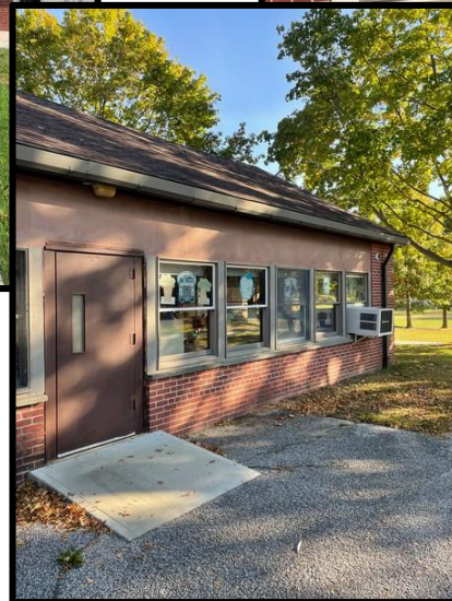
Smithtown Elementary Window Replacement BEFORE
