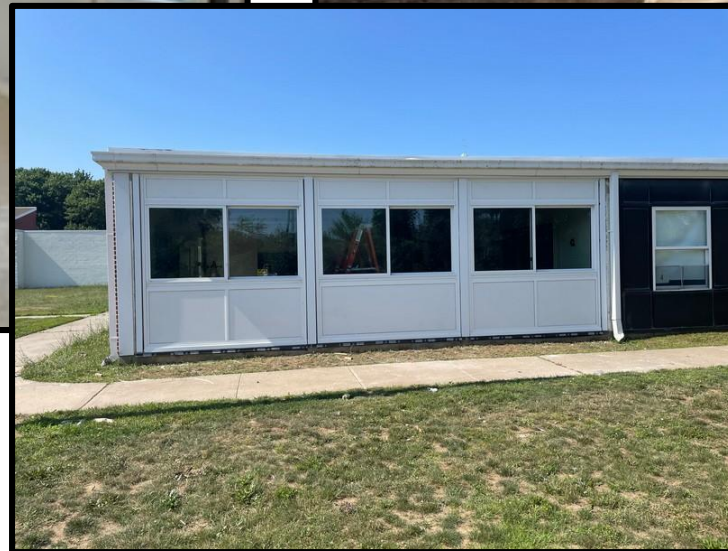
St James Elementary Window Replacement and New Concrete Walkway AFTER
